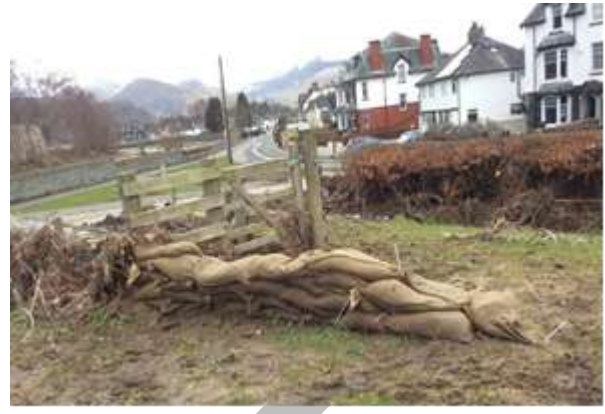
Figure 22 Crosthwaite Road Flood defence wall and embankment which were overtopped
