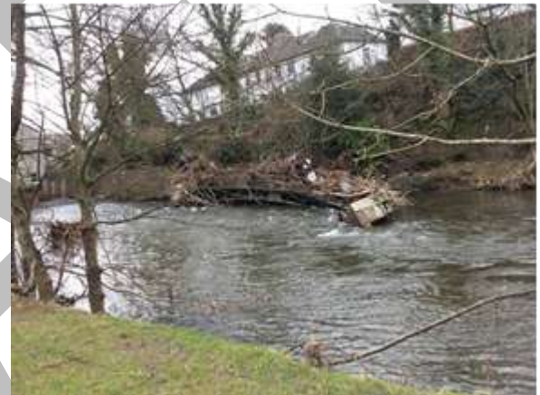
Figure 25 Riverside view of Youth Hostel and washed out footbridge resting on left bank abutment
