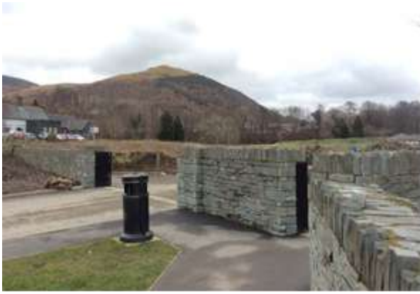
Figure 22 Crosthwaite Road Flood defence wall and embankment which were overtopped
