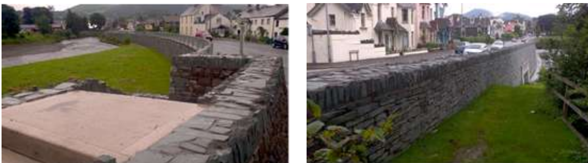
Figure 4 Photos of Keswick Flood Risk Management Scheme - Flood wall along High Hill and Penrith Road
