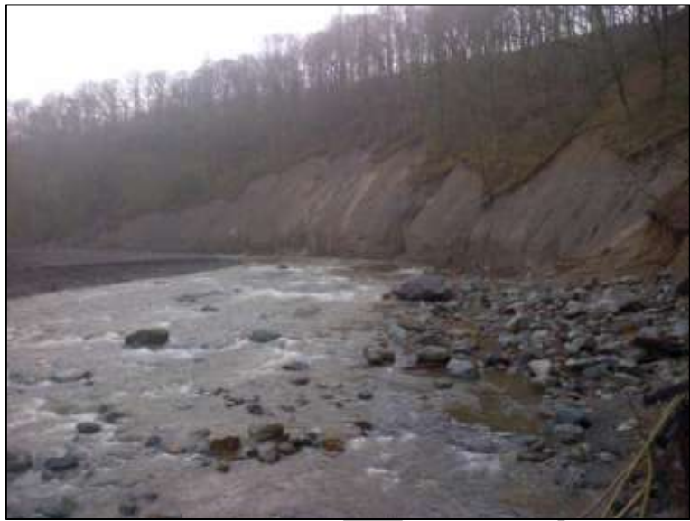
Figure 11 Erosion/landslip feature upstream of Low Briery Holiday Park
