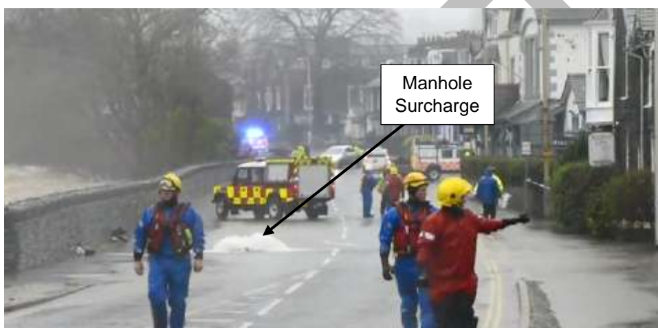
Figure 20 Manhole surcharge on Penrith Road
