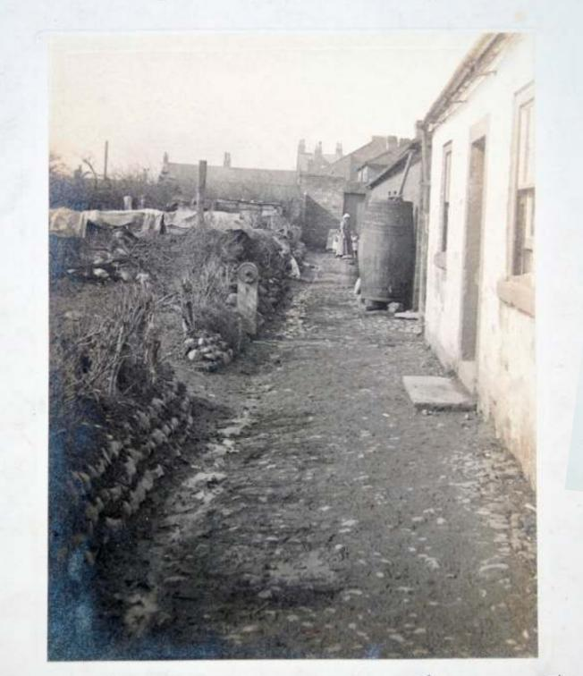
a portion of four houses in California, Kingstown. This property is frequently flooded owing to the absence of gullies in the road; at the rear this road is about 3 feet higher than the house floors, and the only means of carrying away the surface water from this road is by a 4"gully setucied under the water tap shown in this photograph.
