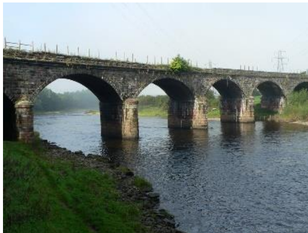
Waverly Line Railway Bridge
