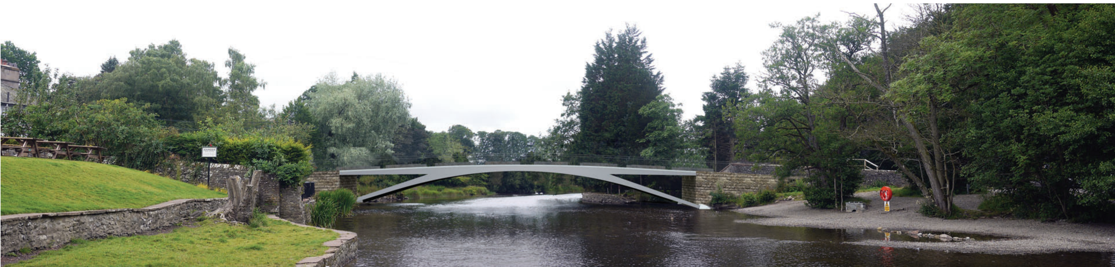
Option C'' | Arched open-spandrel bridge with side structural elements
