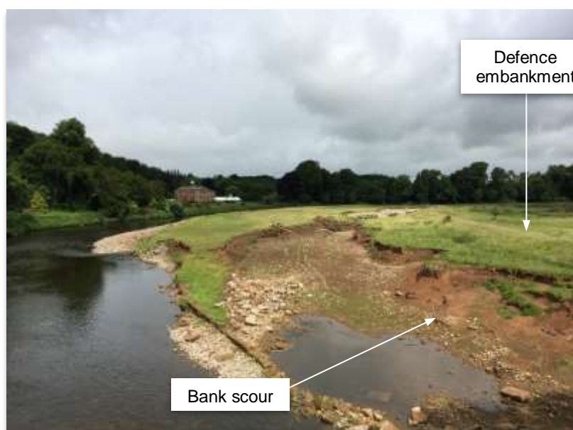
Photograph 6: Scouring to right bank of the River Eden downstream of the A69
