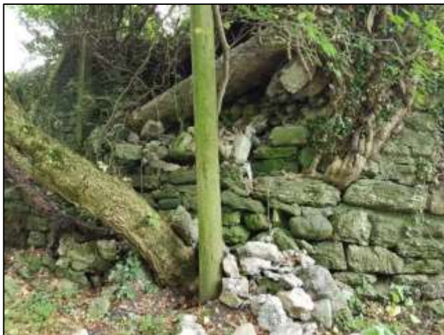
Figure 11: Structural damage on the walls downstream of Beetham Bridge
