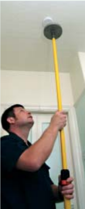
fire alarm testing
