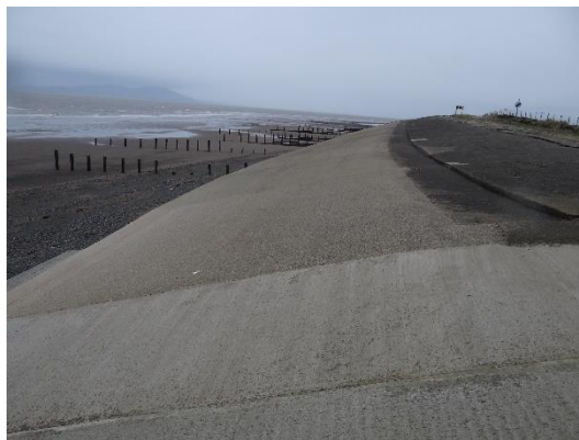
Figure 14 Upper revetment North of Dubmill Scar Photograph taken during CEUK asset inspection (April 2016).
