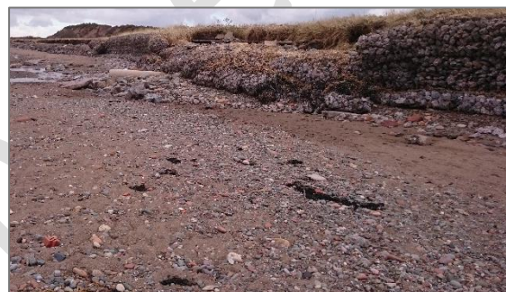
Figure 4 February 2018 - gabion baskets along B5300 North of Maryport Golf Course.
