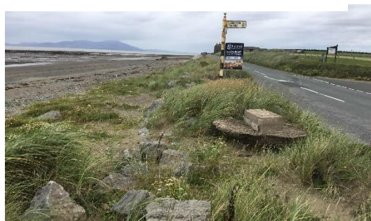
Figure 8 Allonby to Seacroft Farm showing proximity of the highway to the coast. Rock has been placed here to protect the road; occasionally this becomes partially buried by dunes. Photograph taken from CH2M (2017).
