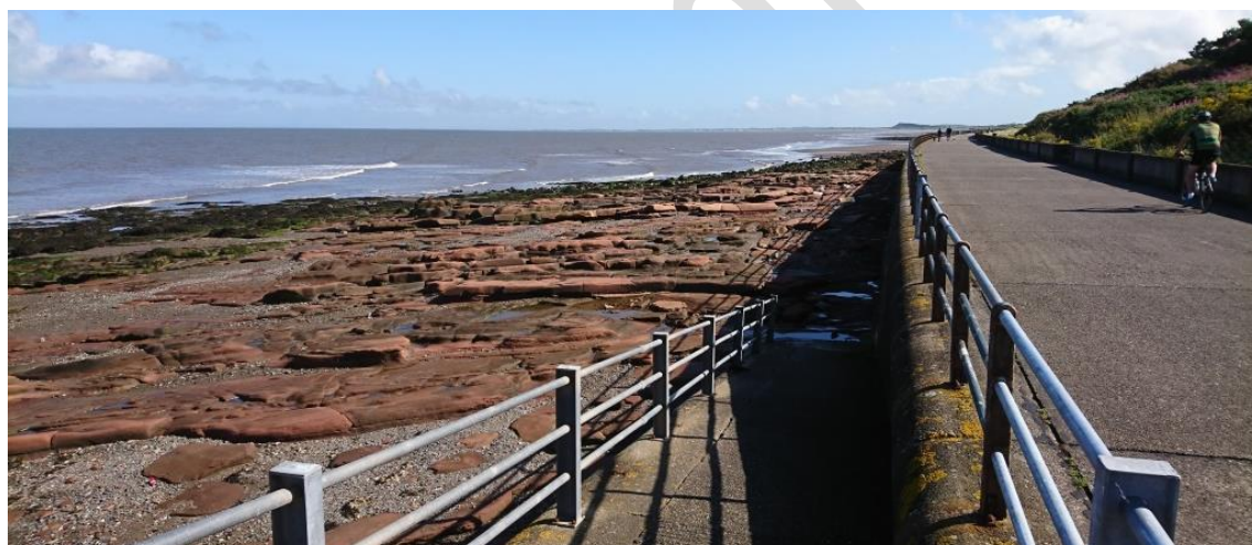
Figure 19 Sandstone bedrock outcrop fronting seawall and cliffs. Photograph taken during CH2M (2017) asset inspection.
