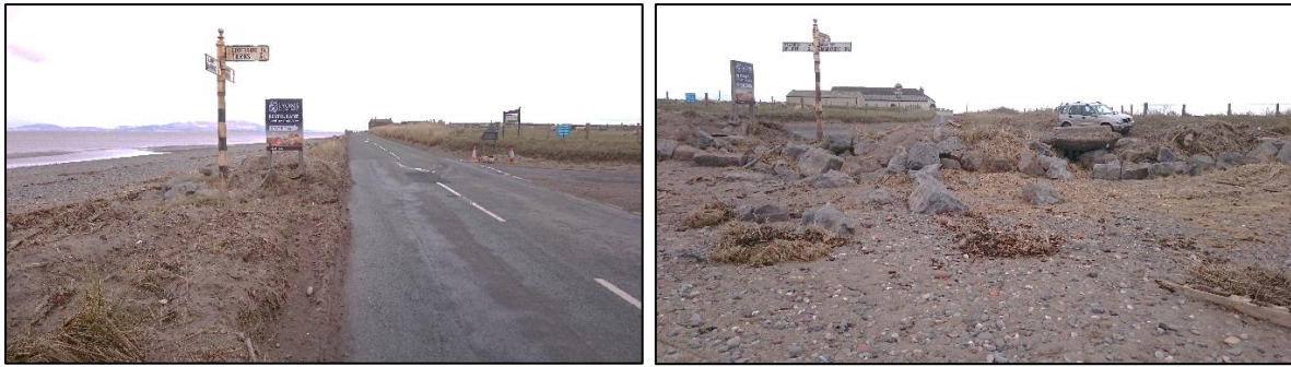
Figure 9 Allonby to Seacroft Farm showing proximity of the highway to the coast. Rock has been placed here to protect the road; occasionally this becomes partially buried by sand. Photograph taken February 2018.
