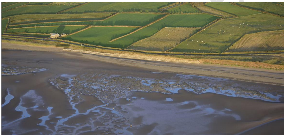
Figure 8 Oblique aerial photograph (2015) showing defences protecting a short stretch of the B5300 at Beckfoot. © Northwest Regional Monitoring Programme.
