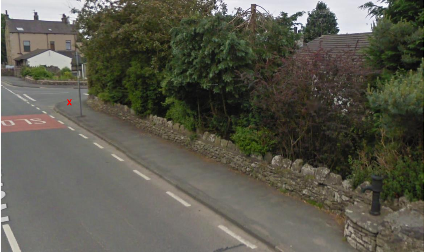
Figure 13: The pump in the bottom right of the picture is now purely ornamental. It is believed to have been moved from approximately the location as indicated by a red X.
