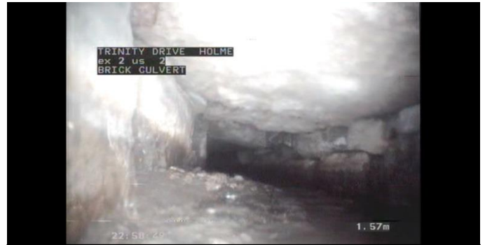
No further progress in upstream direction, low roof and debris shoal directly beneath wall of building restricts clearance and camera can't get through. Significant flow does come through this branch though as seen with dye testing.
