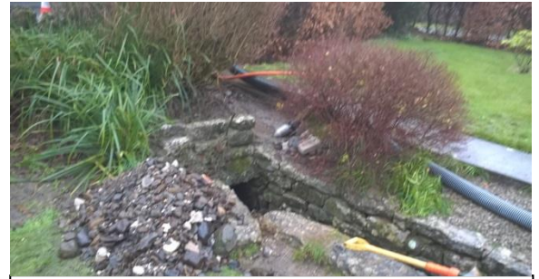
Lots of gravel collects at step down as open channel changes to pipe. CCTV image is looking upstream to waterfall. 450mm dia. concrete pipe.
