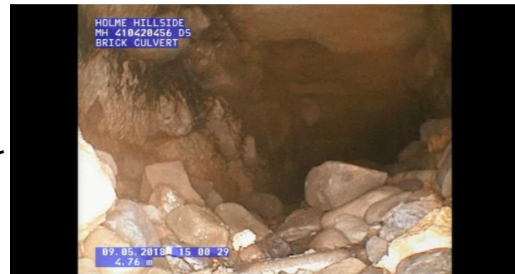
Large stone debris deflects camera into sides. Camera can't pass. This section is recorded as 450mm x 450mm, brick.
