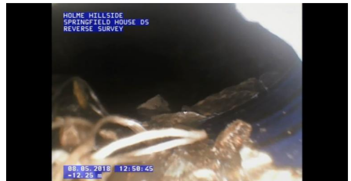
Culvert reduces from 450mm dia. plastic to 300mm x 300mm brick.
