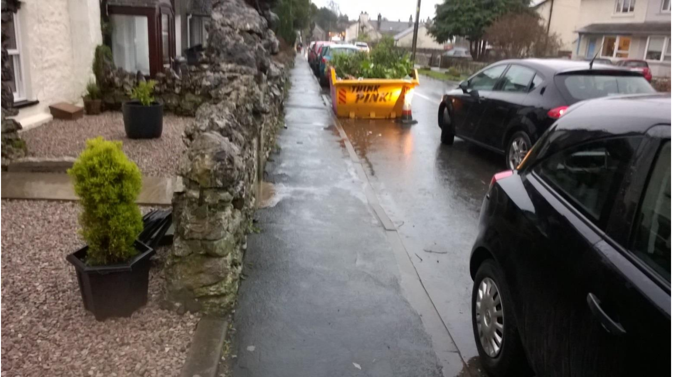
Figure 12: Water pooling upstream of the same skip on North Road during heavy rain on 14 th December 2017. No flooding occurred on 14th December 2017 so it can be assumed that surface flows were much greater during the flood event of 22 nd November 2017.
