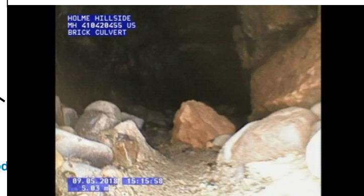
Large stone debris deflects camera into sides. Camera can't pass. This section is recorded as 450mm x 450mm, brick.
