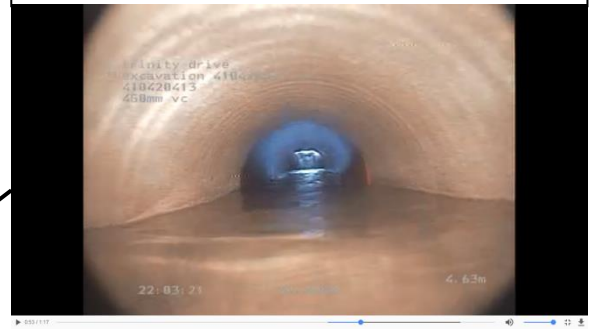
Lots of gravel collects at step down as open channel changes to pipe. CCTV image is looking upstream to waterfall. 450mm dia. concrete pipe.
