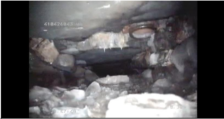
Debris, stones on base from culvert wall.
