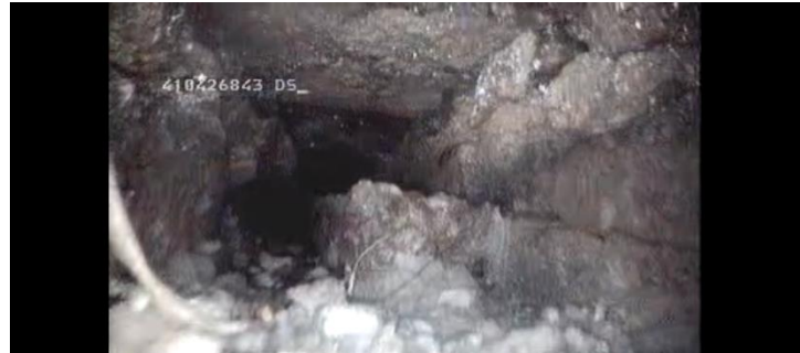
Large brick in the line from side. Where good the dimensions are recorded as 250mm x 250mm, stone.
