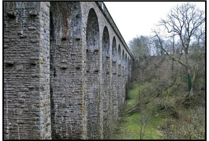
Arches of Podgill viaduct
