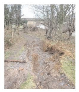
Under the Eden Bridge, at a site visited by the LAF in April 2015, on the path which links the cricket ground with Rickerby Park, a concrete surface has been laid, designed to allow flood water to flow across without damaging the path. Members agreed that hard top paths were a suitable solution in an urban area.
