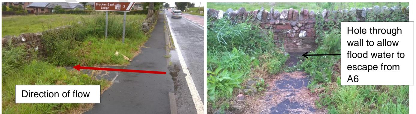
**Photographs 4 & 5: Drainage works to alleviate flooding on the A6**
