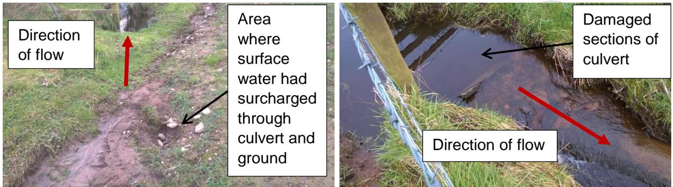
**Photographs 11 & 12: Damage at the downstream end of Brown Sike culvert**
