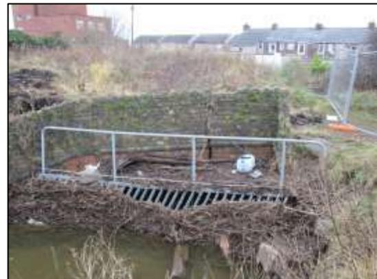
**Figure 23: Risehow Beck grid - erosion on left bank**
