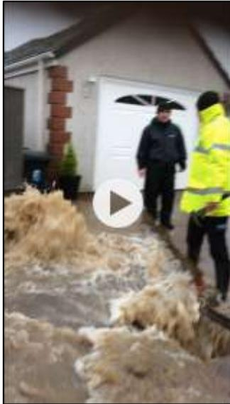
**Figure 10: 6 Allanby Close culvert blockage**
