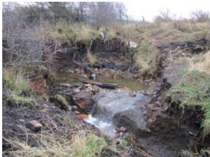
**Figure 24: Erosion behind Risehow Beck grid**
