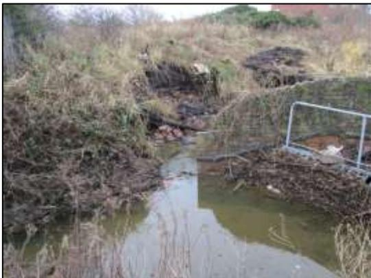
**Figure 22: Risehow Beck grid - erosion on left bank**
