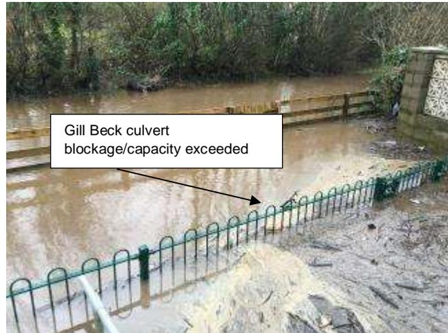
**Photograph 4: Gill Beck culvert - Blocked culvert / capacity exceeded behind Elbra Farm Close**
