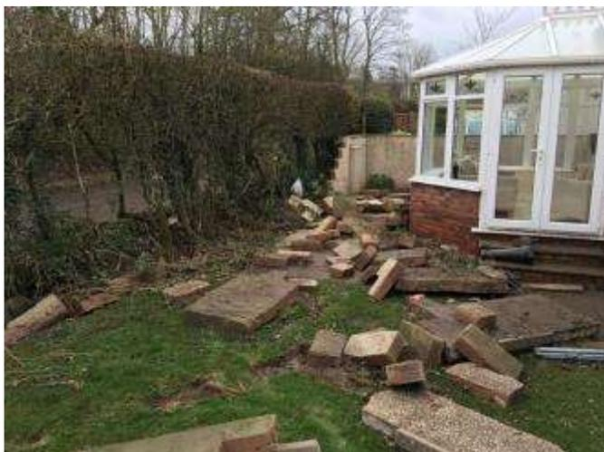
**Photograph 1: Elbra Farm Close – wall destroyed by floodwater**
