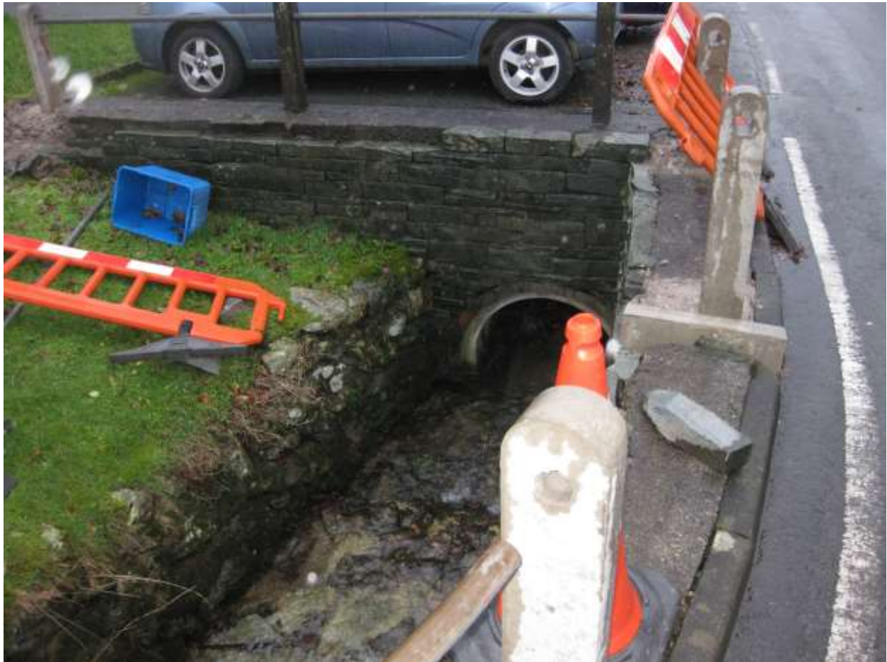
Figure 13 – Culvert on Greenbank Ghyll, which runs parallel to Greenbank Road
