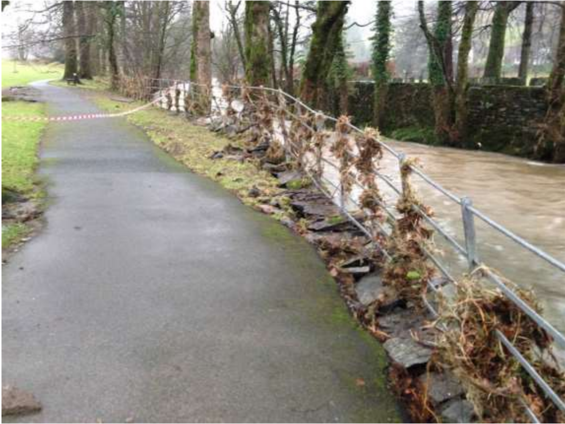
Figure 19 - Flood damage caused by Stock Ghyll in Rothay Park. Note the level of the debris in the railings.
