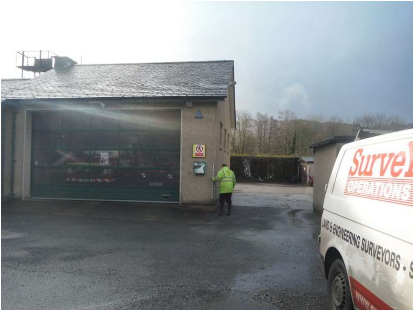
Figure 17 - Recorded water level at the Fire and Rescue Centre
