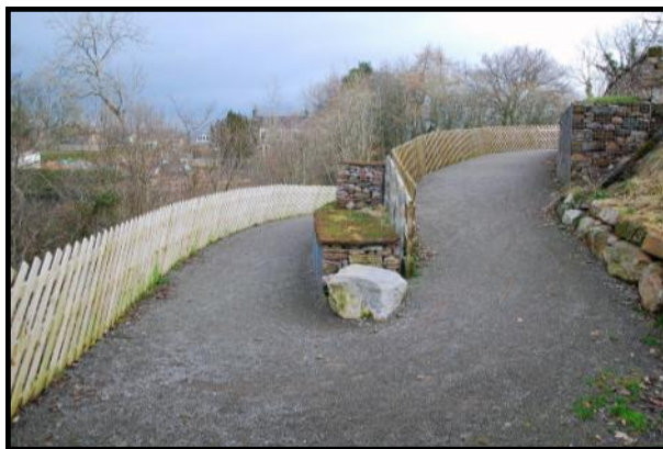
Hairpin bend on the initial section, as viewed from the rest point
