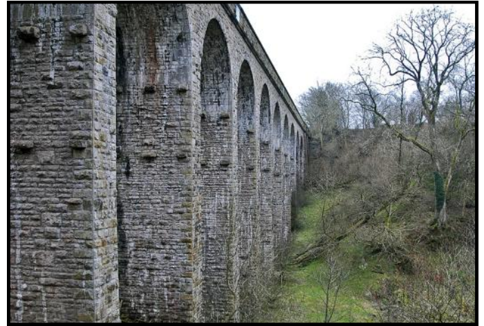
Arches of Podgill viaduct
