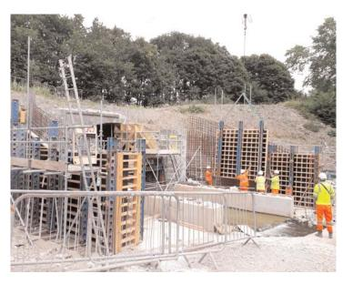
Martin Dean, Site Agent for Kier Construction, explained the ongoing repair work, joint with the Canal and River Trust, to rebuild the aqueduct. The original stones have been numbered and will be reused.
