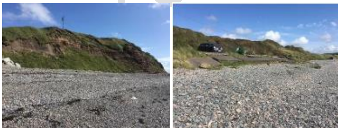
Figure 9 Nethertown 2 – Natural Cliff and Slipway at Nethertown shore car park (11d5.5)
