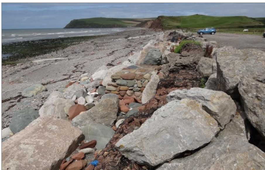
Figure 15 Sea Mill (North of Ancient Fishgarth) - Rock revetment and gabions
