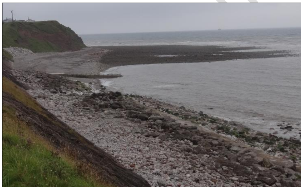
Figure 13 11d5.6 (Coulderton to Sea Mill) - various defences
