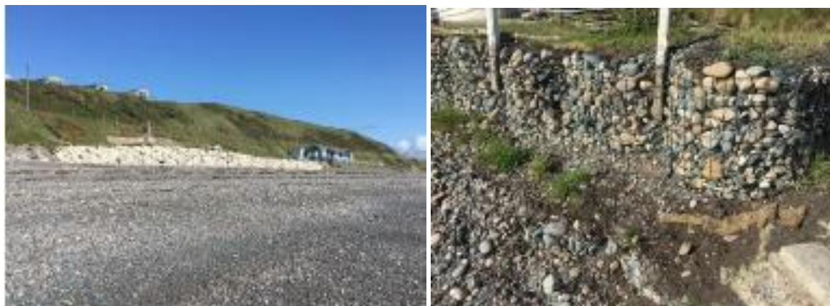
Figure 8 Braystones – rock revetment and gabions
