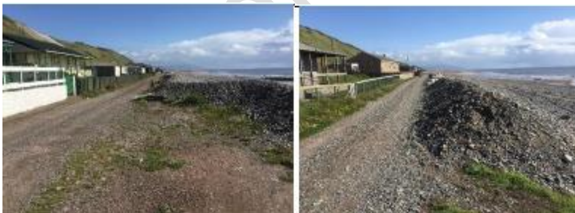
Figure 11 Braystones to Coulderton – shingle beach reprofiling
