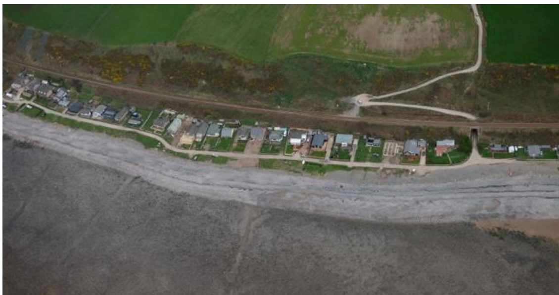
Figure 10 Coulderton – beach properties (11d5.5 and 11d5.6) © North West Regional Monitoring Programme, 2015
