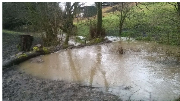
Figures 13 and 14: Leaky dams; some of the measures used in the Stroud rural sustainable drainage project
