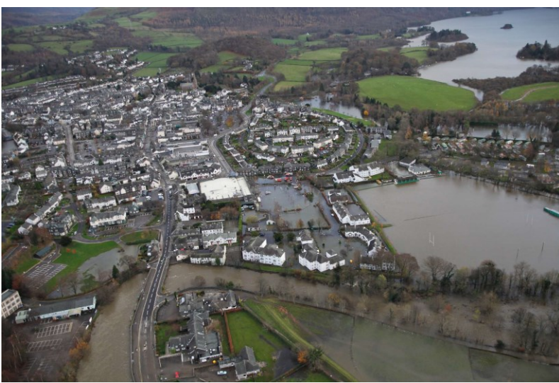
Figure 9: Photograph of flooding in Keswick, Cumbria during the winter 2015 floods
