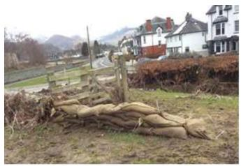
Photograph 31: Crosthwaite Road flood defence embankment that was overtopped
