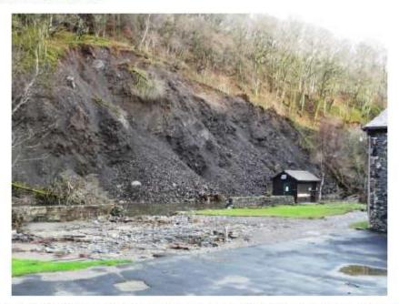
Figure 11: Part of the bottom of the Brundholme woods slope where the river has eroded the bottom of the slope (the brown hut is the EA gauging station).
