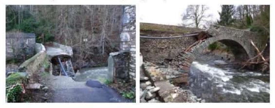
Figure 12: Damage to bridge in The Forge area.
