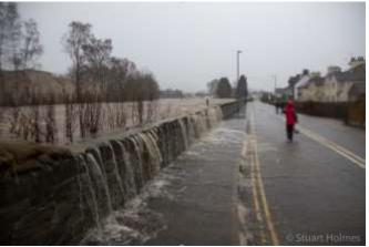
Photograph 33: Overtopping of flood defences on Crosthwaite Road
