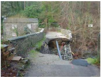
Photograph 6: Forge Bridge Partially Collapsed
