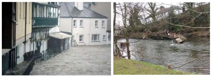
Photographs 18 and 19: Riverside view of Youth Hostel (left) and washed out footbridge resting on left bank abutment (right)
