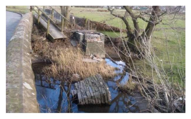
Photograph 3: Damaged storm water bridge, Howrahs
