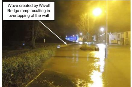
Photograph 13: Wave created by the access ramp on the left bank at Wivell Bridge Cumbria.gov.uk
