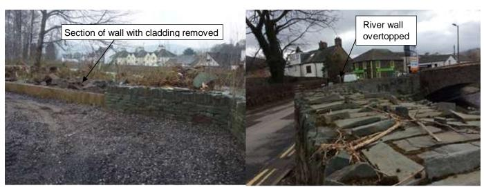
Photographs 20 and 21: River overtopped its bank/flood wall at Southey Hill Estate (left) and the river wall overtopped at upstream of Greta Bridge (right)
