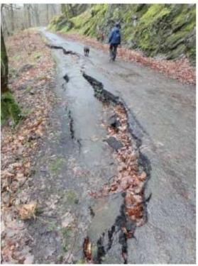
Figure 10: The top of the Brundholme Woods landslip visible in the minor road through the woods.
