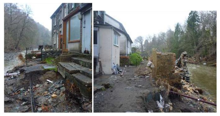
Photographs 7 and 8: Scour damage to the rear of properties
