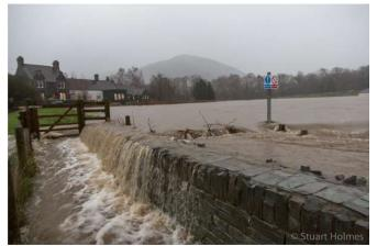
Photograph 32: Overtopping of flood defences on Crosthwaite Road
